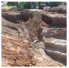
Vitrified clay pipes are traditionally used in this region on account of this material's outstanding abrasion resistance and long service life. Given the high density of underground supply pipes, pipe sections of short length were mainly used for this project.
