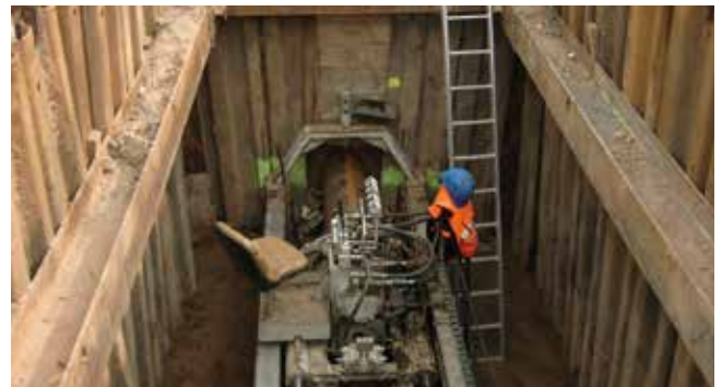
Sheet pile lining
