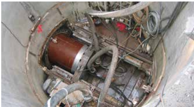
Reinforced concrete sinking shaft
