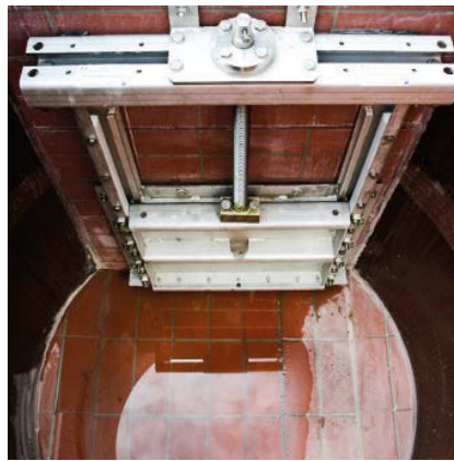
Gate-valve installation
