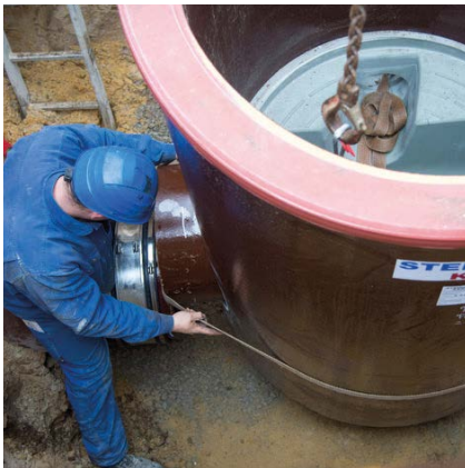
Setting the manhole in place
